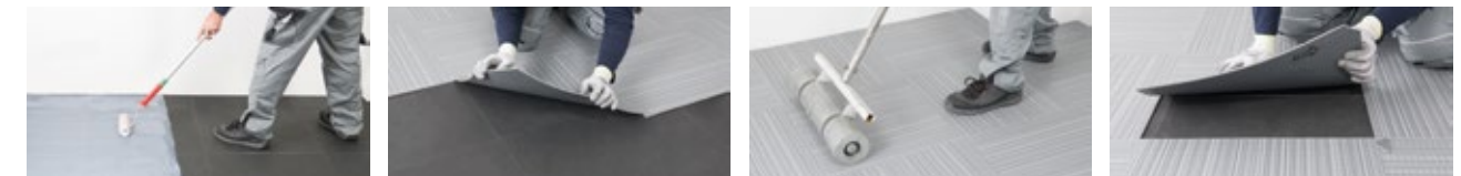
Installation with tackifier
