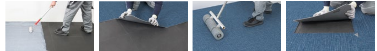
Installation with tackifier
